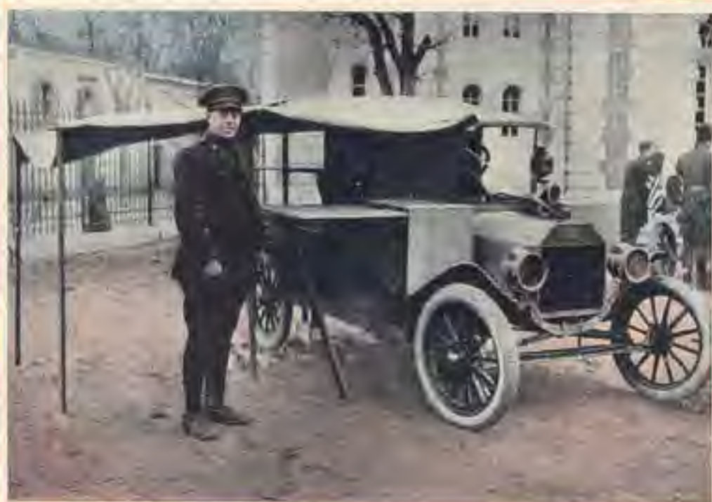
Ford supply and repair car with canvas side extended to form a roof and sides of lockers raised to form a workshop
